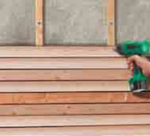
Assembly of the facade cladding
